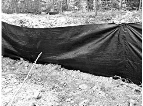
Silt Fence: A BMP used commonly in Pike County to control soil sediment on earth disturbance sites
